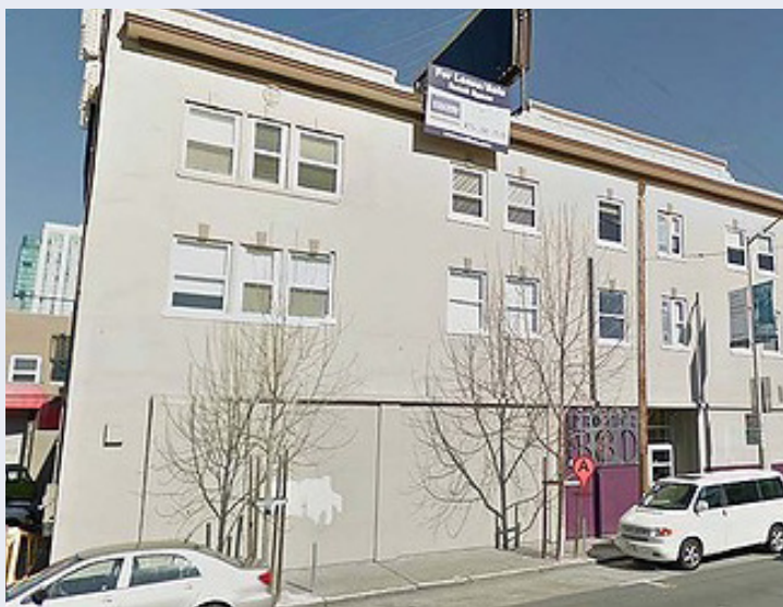
StartUpHouse - Google Street View
