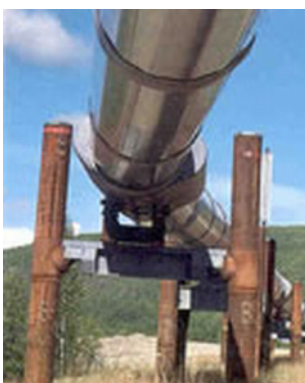
Ethanol's corrosive properties could pose problems for the transportation through pipelines.
