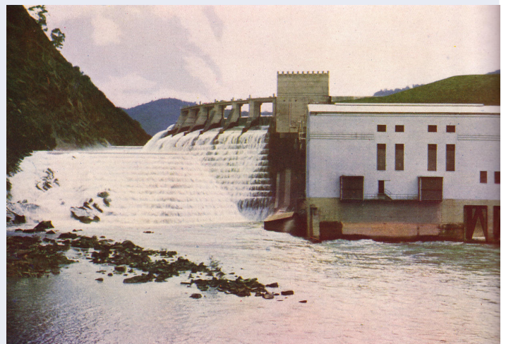
Sugarloaf Power Station, below the Eildon Weir Spillway, part of the Rubicon Hydroelectric Scheme
